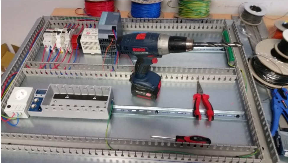
Fig 17 : rails fixation, components mounting on the supports and cabling
